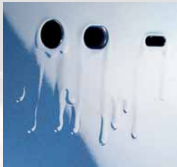
Removing paint runs
